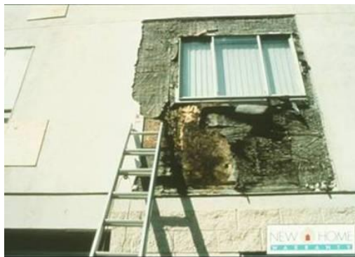
Figure 1: Examples of building damage due to improper flashing and installation. The figure on the left shows damage that occurs behind the building façade, while the picture on the right shows damage at the interior sill of the window.
