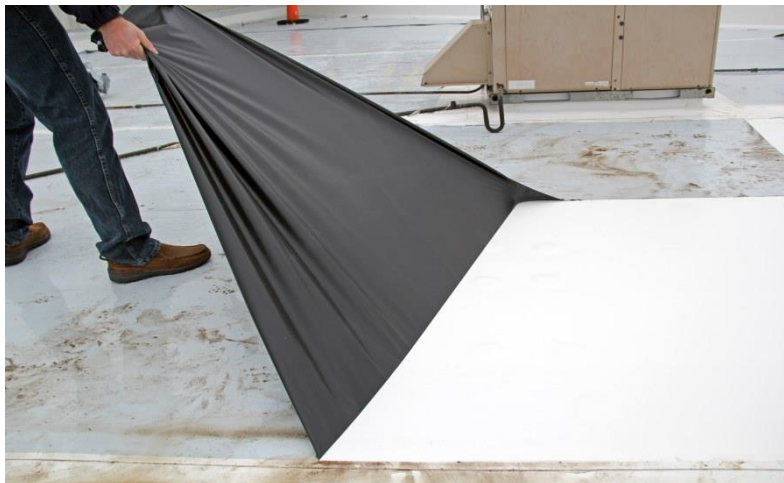
Figure 7 . Protective liner being removed from a completed thermoplastic roof.
